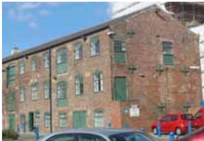
A former flax warehouse to Marshall's Mill. The first of Marshall's buildings south of the Holbeck dating from 1808 and the first of his buildings to use the cast-iron column and beam and brick arch system. Well restored to provide modern offices.
